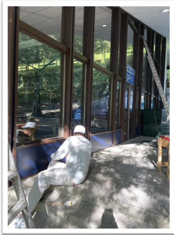
Thanks to our WVSD team for painting our panels.
